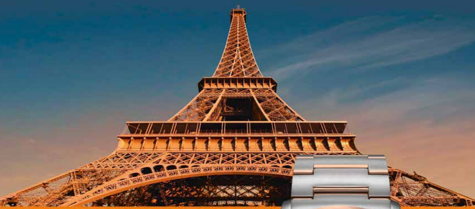
Eiffel Tower, Paris France
